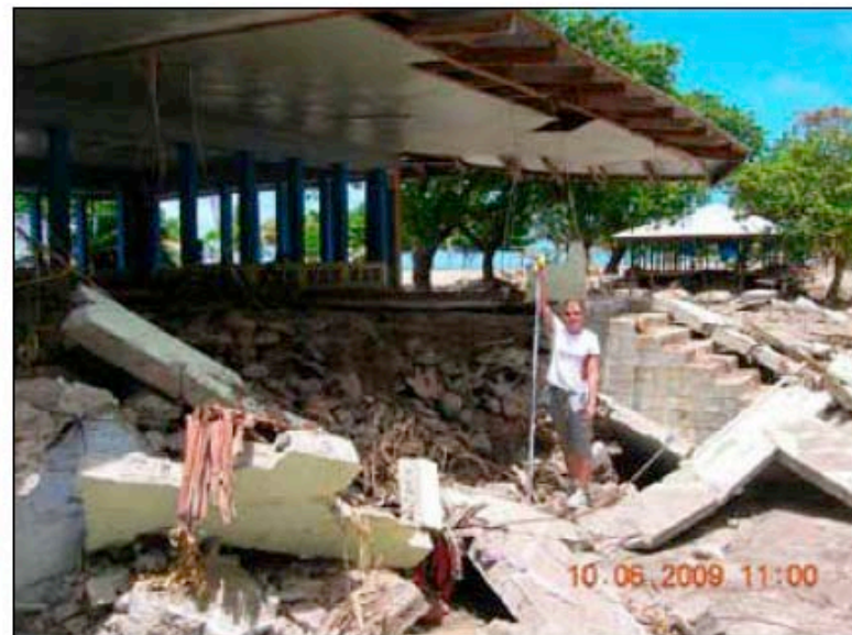
Figure 8. In Lepa, Samoa, scour caused the collapse of part of a village meetinghouse.
