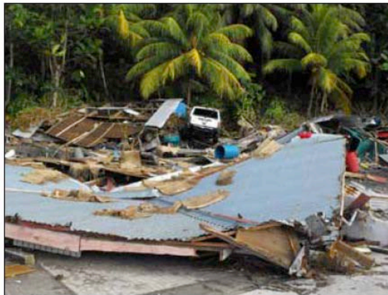
Figure 6. Debris piled up at more than 12 m elevation at Poloa, American Samoa.
