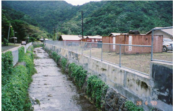
Picture 6 PDM Flood Control Project. Mitigation for chronic flooding to LBJ Hospital
