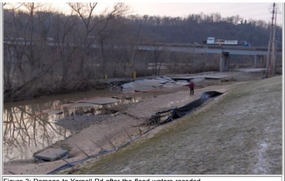
Figure 3: Damage to Yarnell Rd after the flood waters receded
