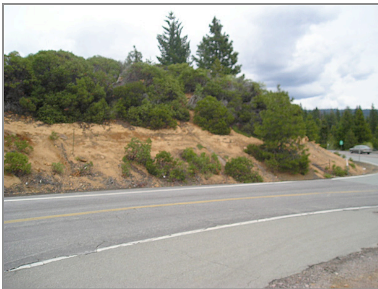
Figure 10. A roadcut exposing > 2m thick deposits of the Big Canyon Creek lahar in the study area.
