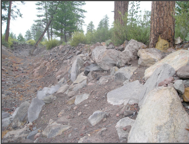
Figure 7. Photo of Whitney Creek, right bank boulder levee downstream from the US97 culvert. Scarring on buried pines indicates peak flow depth.
