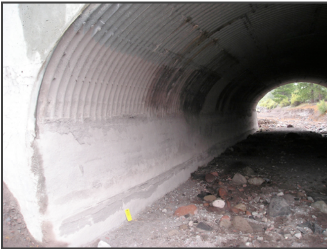
Figure 8. Mud lines as seen in the US97 culvert indicating the height of wave crests during the 1997 Whitney Creek debris flow.
