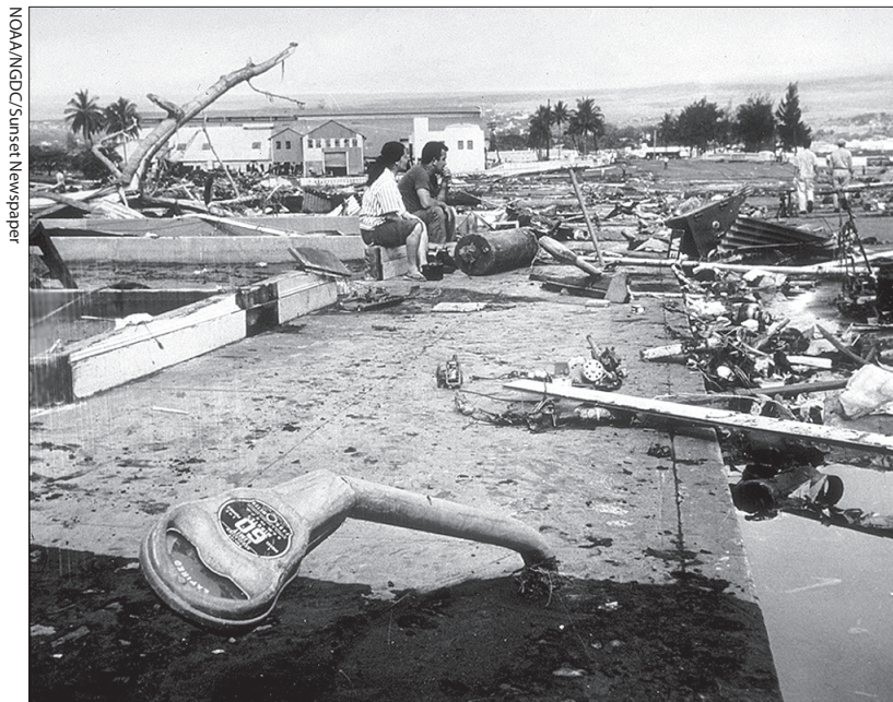
A major earthquake off the coast of Chile on May 22, 1960 produced a tsunami that affected the entire Pacific Basin. In Hilo, Hawaii — 10,000 km from the earthquake — the tsunami caused 61 deaths and $24 million in property damage. Frame buildings were either crushed or floated off their foundations, and only buildings of reinforced concrete or structural steel remained standing.
