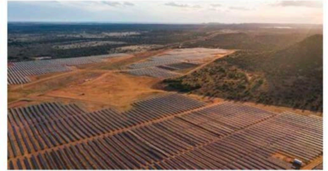
The Holstein solar project in Texas during construction. Image: 8minute Solar Energy
