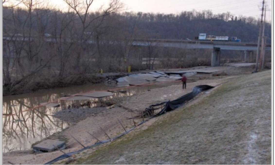
Figure 3: Damage to Yarnell Rd after the flood waters receded
